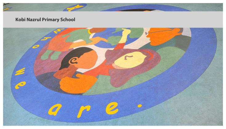
A spectacular flooring design chosen by pupils has been cut from Marmoleum, using Forbo Flooring Systems' unique Aquajet Technology.
